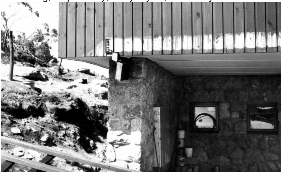
At original entrance-today the switchboard downstairs
